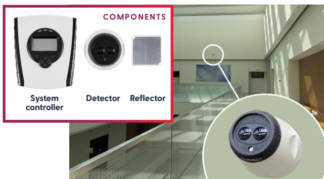
FFE's Fireray® 5000 system protecting the courthouse atrium
