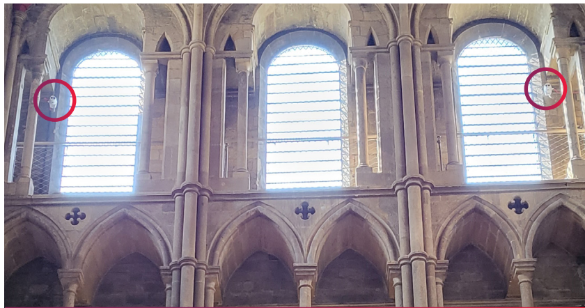
Beams mounted close to windows in the transept
